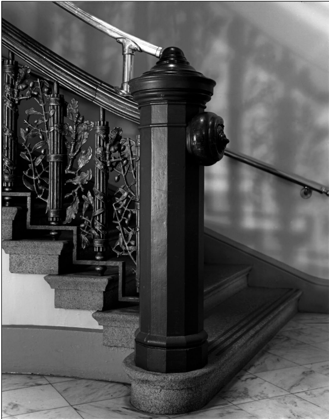
Stairway Ironwork in the Treasury Building, Washington, DC
