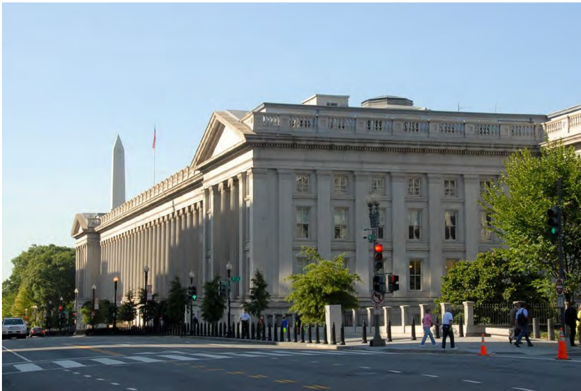
Figure 1: Main Treasury Building in Washington, D.C.
