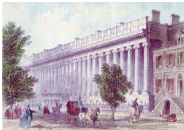
▲ East front of the Main Treasury circa 1865. The 336-foot long colonnade was rebuilt with granite in 1908. On the right stands the old State Department building, which was razed in 1866 to make room for the north wing of Main Treasury.
